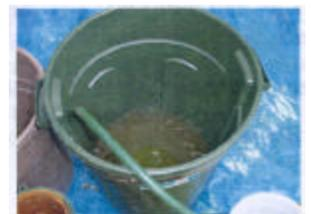
Be aware that some solid chlorine products used for swimming pools may have additional chemicals, such as algacides, in them and should not be used for well disinfection. Place the can next to the well to pour the solution or siphon the chlorine solution from the can to the well.
